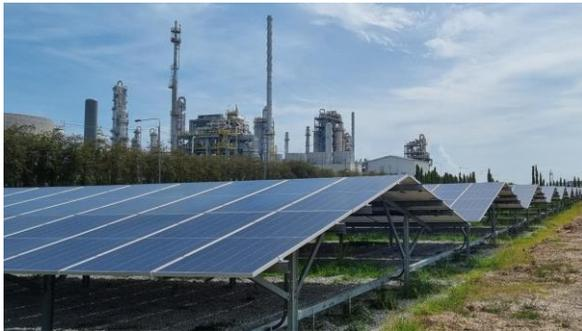
In partnership with Glow, Indorama Petrochem Limited (PTA) completed the installation of ground-mounted and rooftop solar panels at the site in 2022, with a total capacity of 2.96 MWp. The solar panels are expected to generate 4,500 MWh/year, contributing to an annual reduction of 1,800 tCO<sub>2</sub> in GHG emissions
