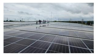
In 2022, Petform (Thailand) Limited in Nakhon Ratchasima installed a new solar plant with a capacity of 586 kWp, contributing to an annual reduction of 351 tCO<sub>2</sub>e in GHG emissions.
